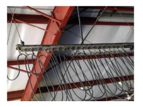
For large cover production festoon systems are a neat solution for cable management. A festoon system consists simply of mobile hangers on a suspended trackway that can move the welder's power supply cable as the welder moves below during welding.
